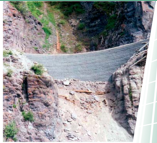
Collins' California office was responsible for the design of a welded wire retaining wall to replace a failed timber wall in Telluride, Colorado for San Miguel County. The structure measured 24 feet high at its maximum.
