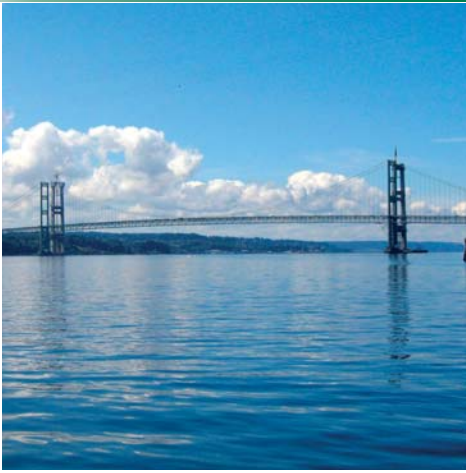
Since 1996, Collins has provided underwater inspection and assessment services of over 200 bridge structures for the Washington State Department of Transportation. Most recently, the bridges inspected have included multi-span structures with up to 15 spans, as well as floating bridges. Inspection efforts have included diving to water depths of up to 145 feet, and the use of ROVs with real time video documentation at greater water depths.
