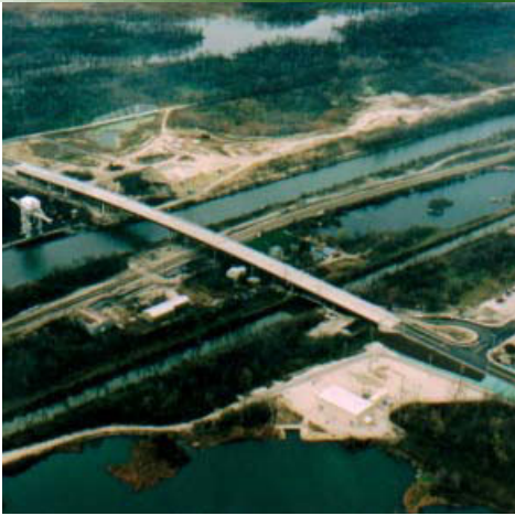
Collins was retained to design a high level bridge over the Chicago Sanitary and Ship Canal, the BNSF Railroad, and the Illinois and Michigan Canal.
