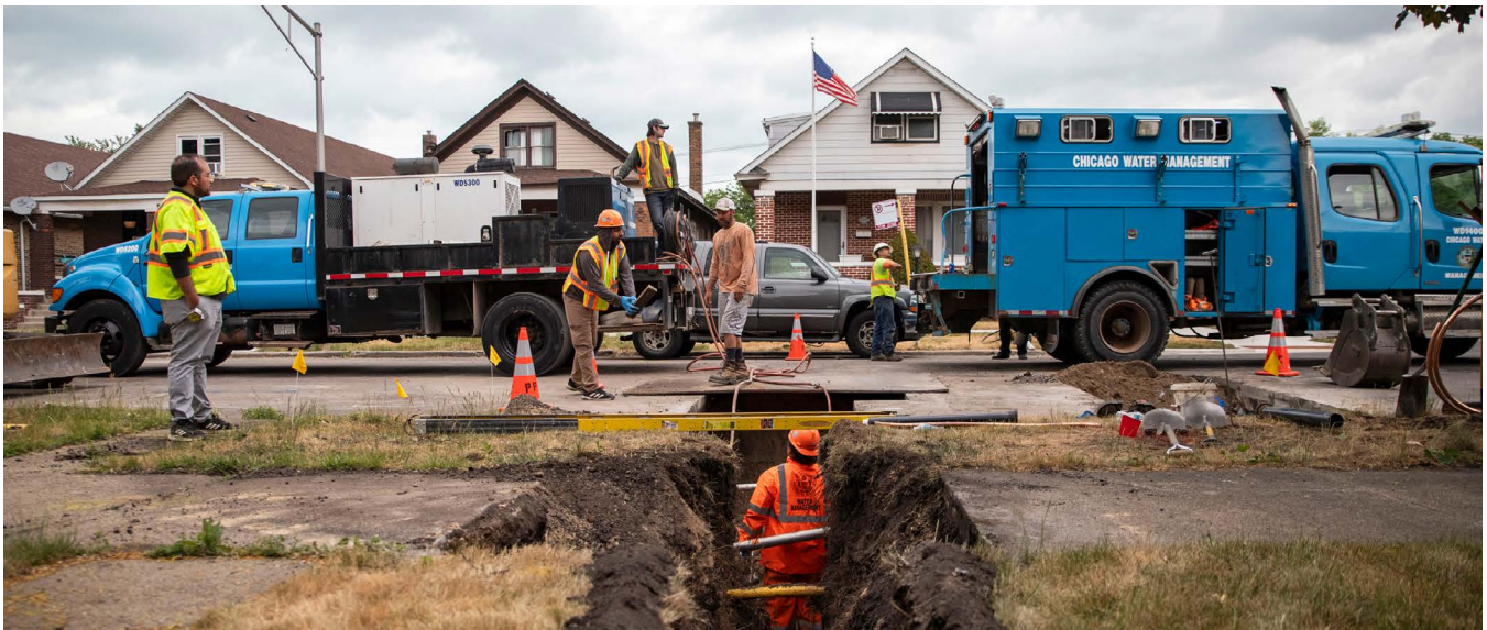
Lead service line replacement (NRDC, 2024)
