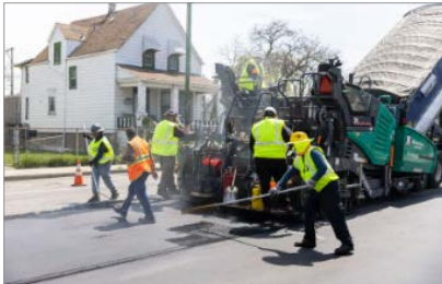
CDOT construction crews resurfacing street with asphalt
